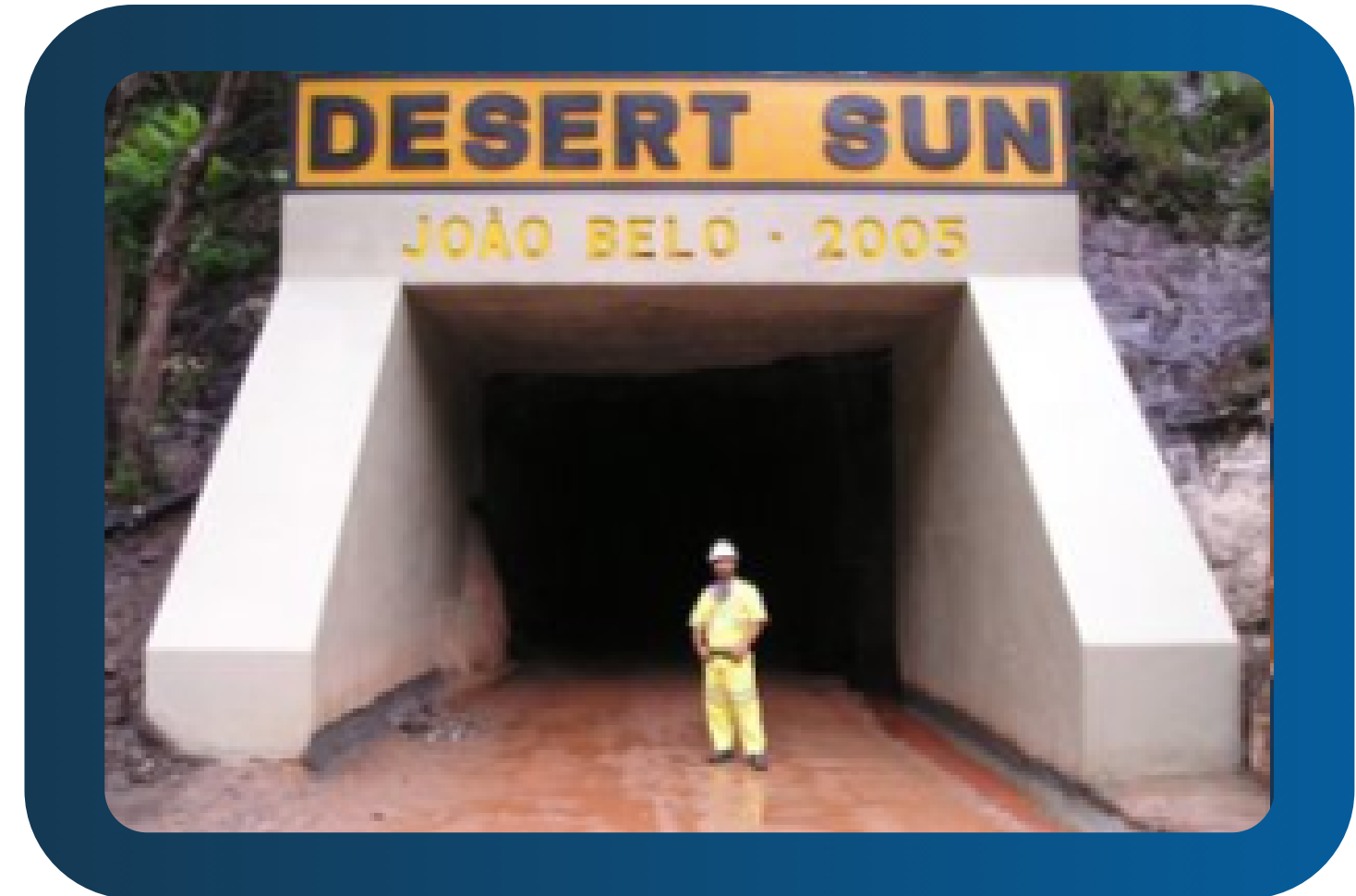
Finished mine access portal (same access portal)
